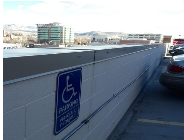
Fourth Floor Barrier – North Facing
