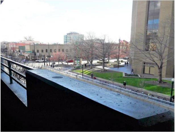
Third Floor Railing – South Facing
