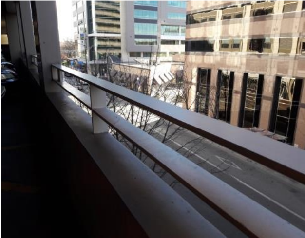
Third Floor Railing – South Facing
