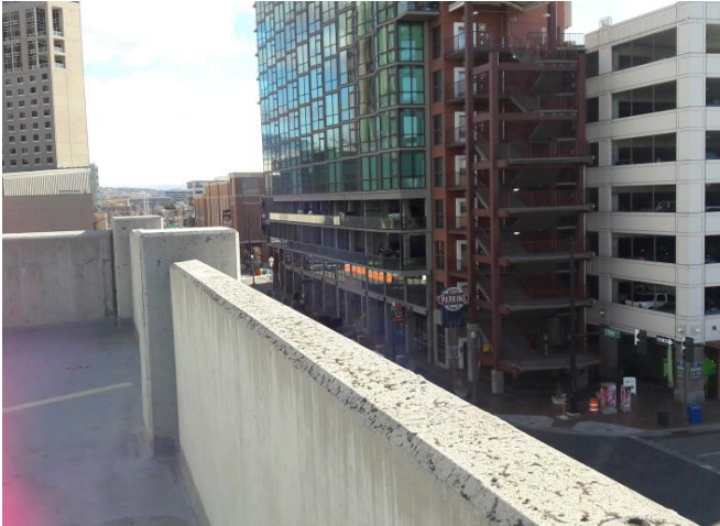
Fifth Floor Barrier – South East Facing
