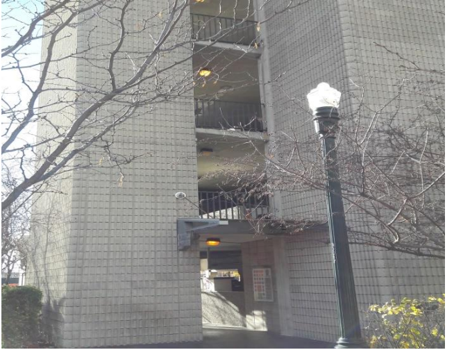
Stairwell / Elevator Exterior
