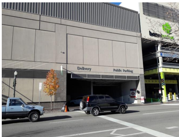
Boulevard Garage Entrance – East Side
