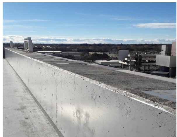
Eighth Floor Barrier – West Facing
