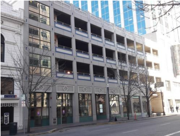
Eastman Garage Front – North Side
