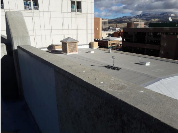
Sixth Floor – East Facing
