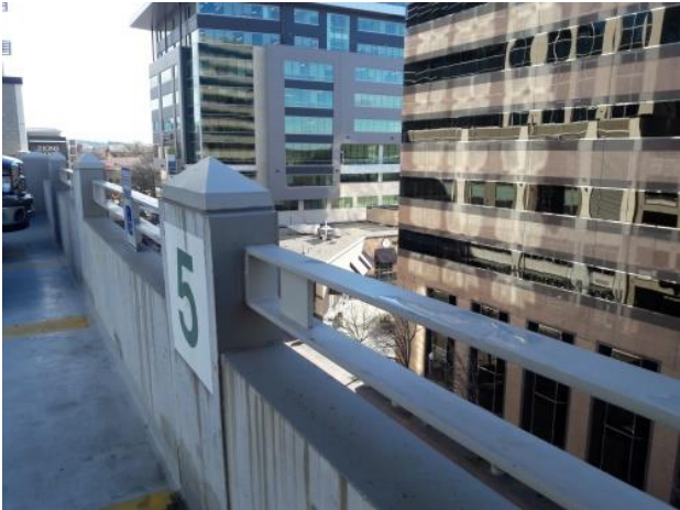
Fifth Floor Railing – South Facing
