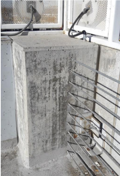
Eighth Floor – Northwest Corner
