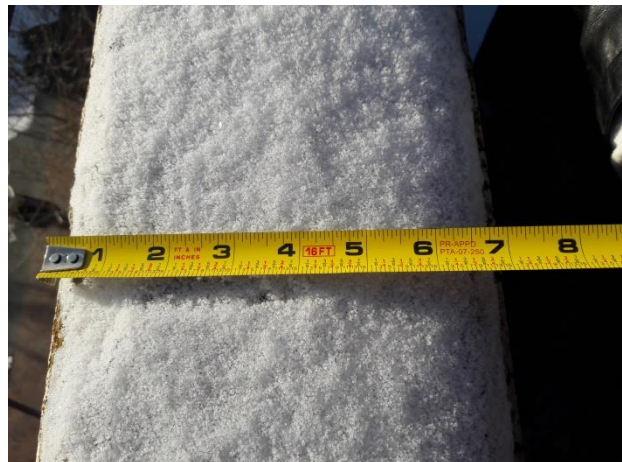
Third Floor Barrier – North Facing
