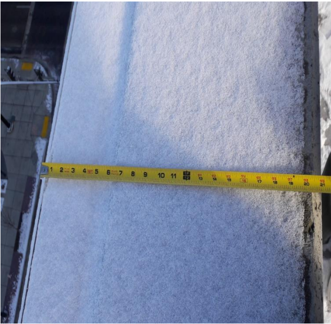
Eighth Floor Barrier
